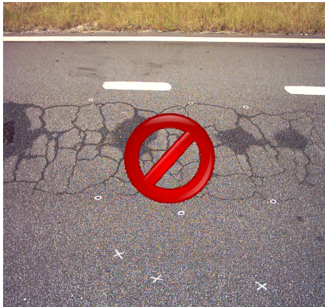
Alligator/Fatigue Cracking
