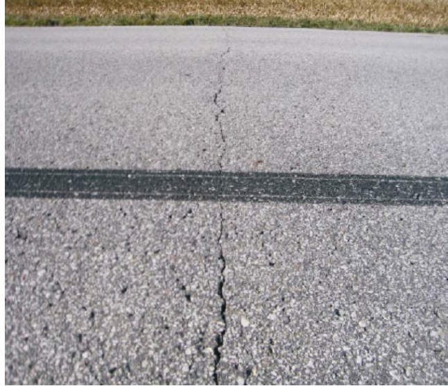
Low temperature cracking
