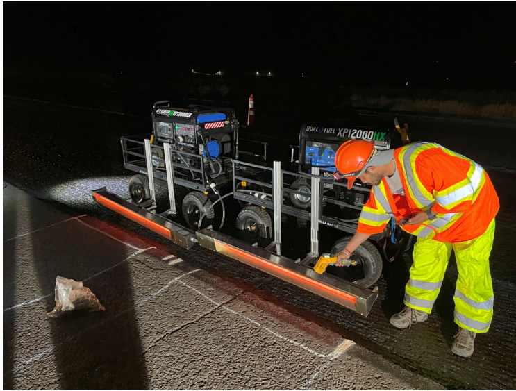
Infrared heating of the joint
