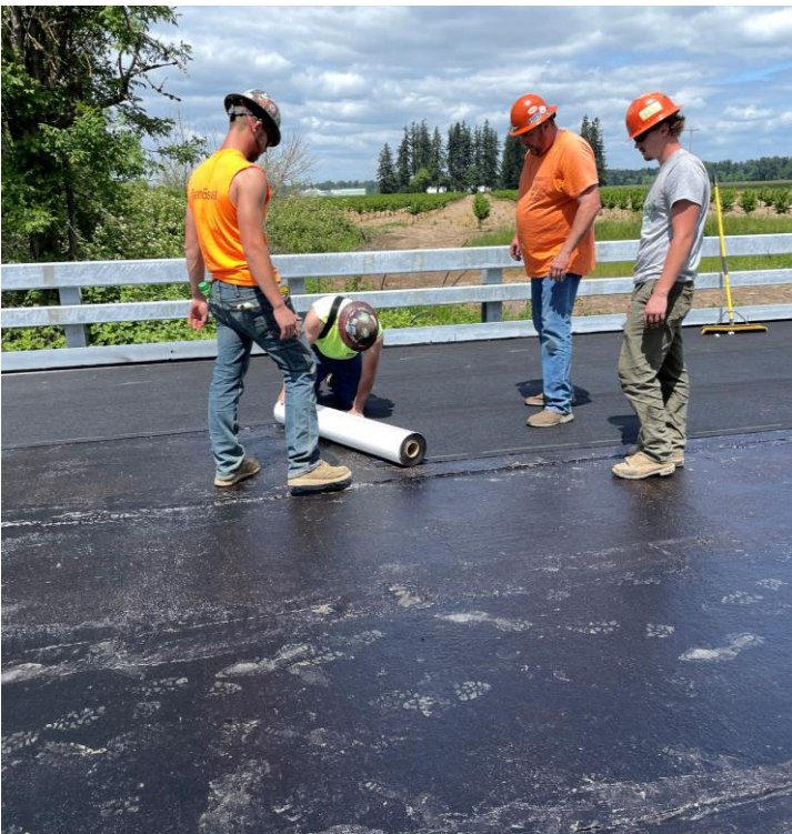
Working towards the Center
