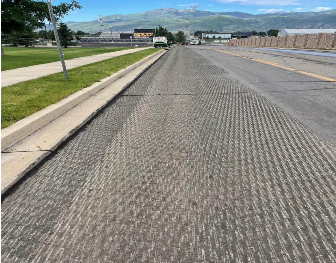
Edge Milling and Installation of Paving Grid Using PG58-28 Binder
