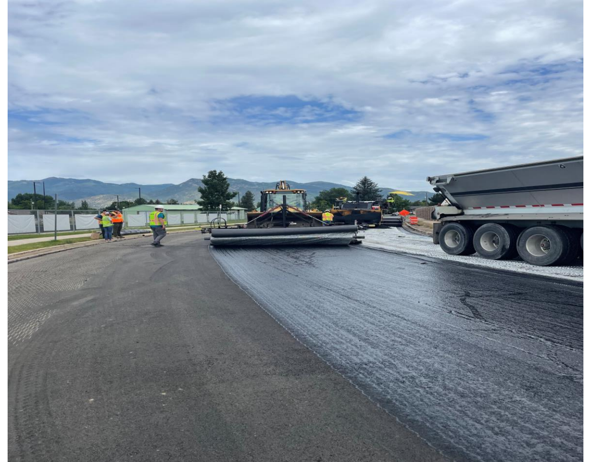
Edge Milling and Installation of Paving Grid Using PG58-28 Binder
