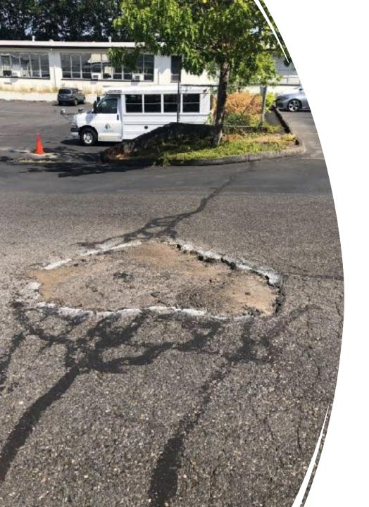
UV Rays, air and water lead to asphalt binder oxidation.
