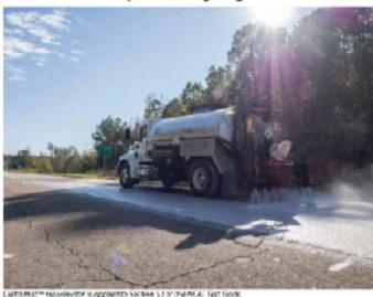
A rejuvenating fog seal is a type of pavement. preservation treatment applied to an existing asphalt pavement surface to preserve its functional and structural integrity and delay. a more costly rehabilitation treatment in the neorfuture.
