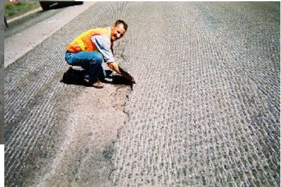
Delamination
