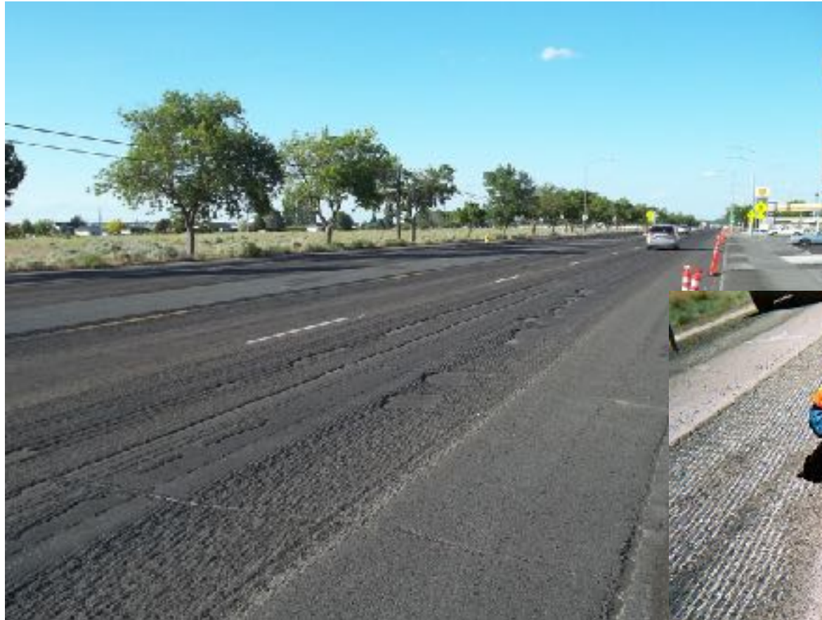
Delamination
