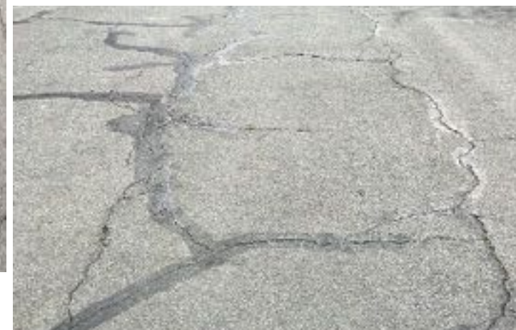
Block Cracking
