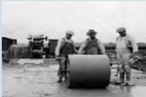
Early 1940s: The first RCC pavement in North America is an airport runway constructed in Yakima, Washington.
