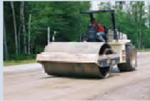
1970s: RCC pavements become common for log-sorting yards in Canada.
