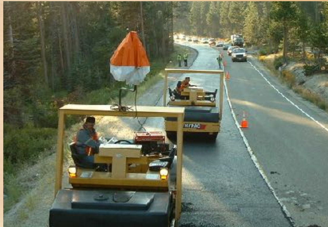
Rolling operation showing traffic control.
