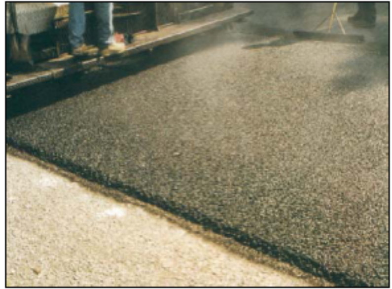
Figure 5: Freshly Laid BWC (11)
