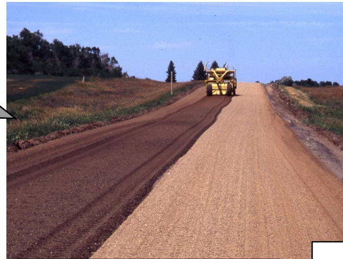
Newly converted road
