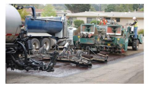
**Sand Seal** is a sprayed application of asphalt emulsion followed immediately by a covering of clean sand or fine aggregate.
