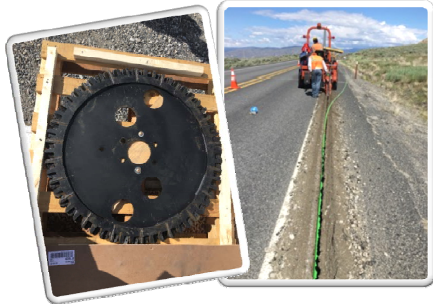
Micro Trenching / Narrow Slot
