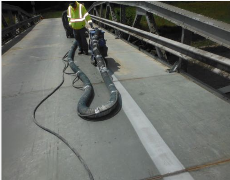
Step 1 Deck Preparation
