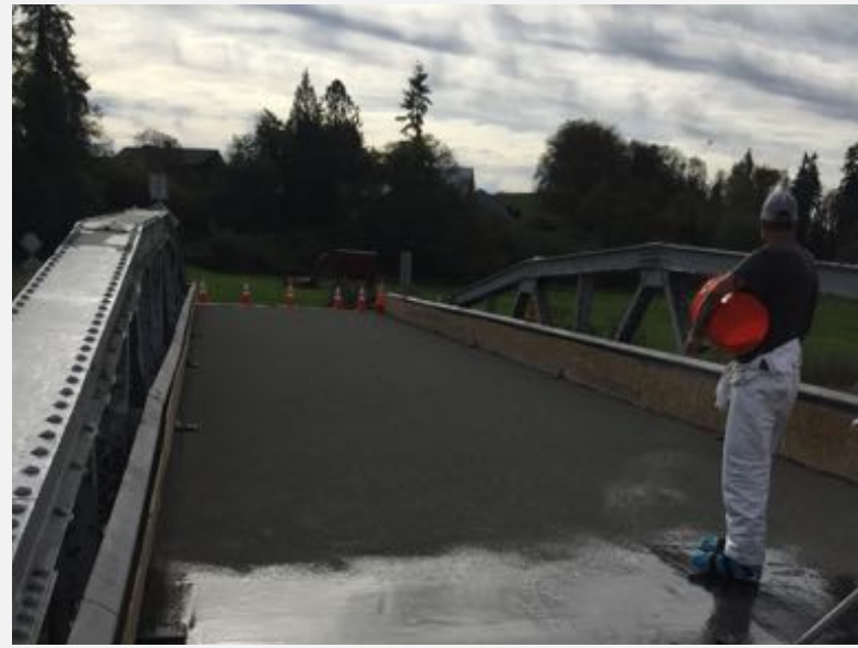
Step 4 Broadcast Aggregate
