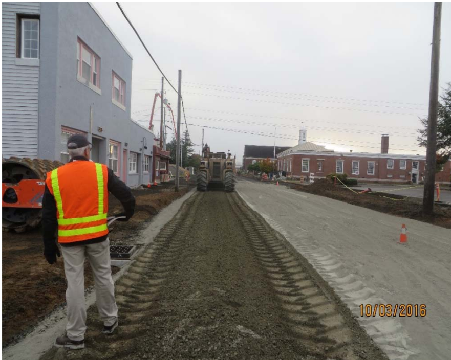
Soil-Cement Stabilized Surface after first pulverization on Duryea Street
