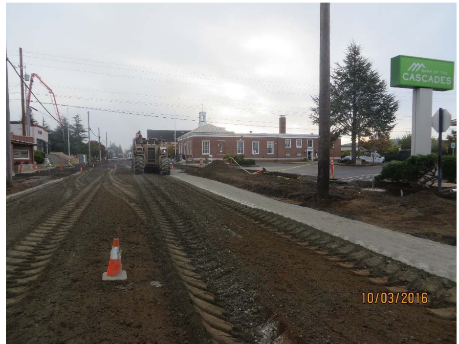
Soil-Cement Stabilized Surface after first pulverization on Duryea Street
