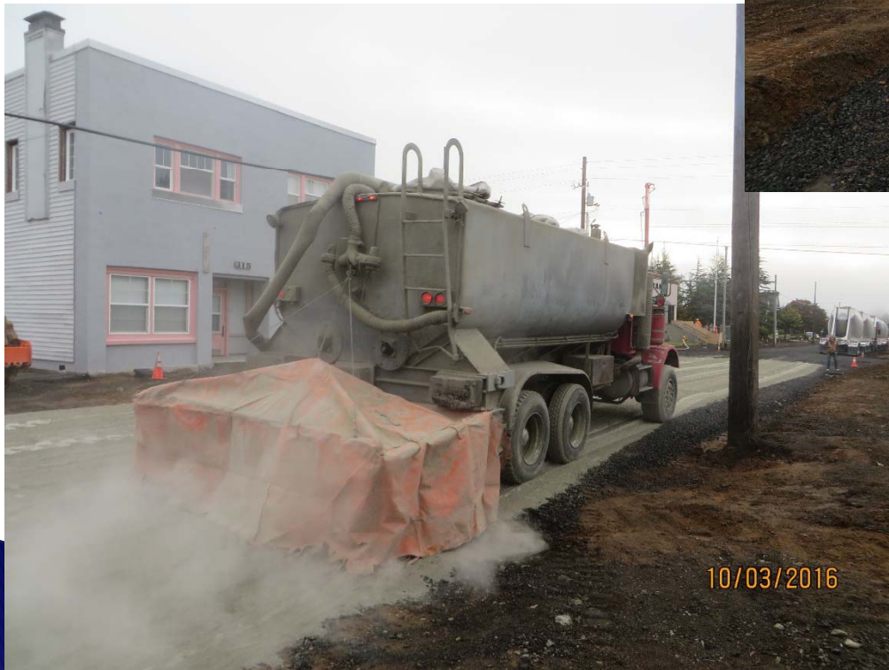
Application of cement to the Soil-Crushed Aggregate blend on Duryea Street October 3, 2016
