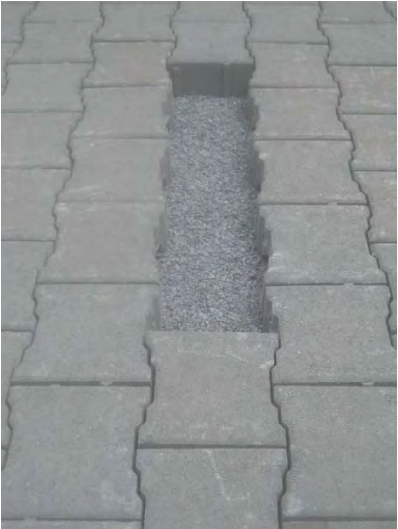
PaveDrain "Lock Blocks" being placed by hand.
