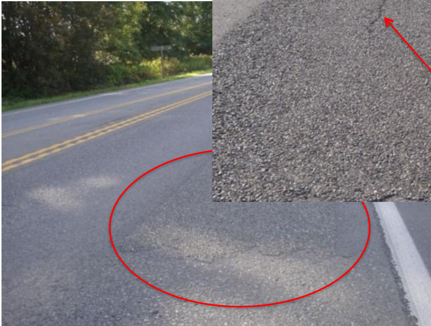
Wheel path chip seal after 1 year.
