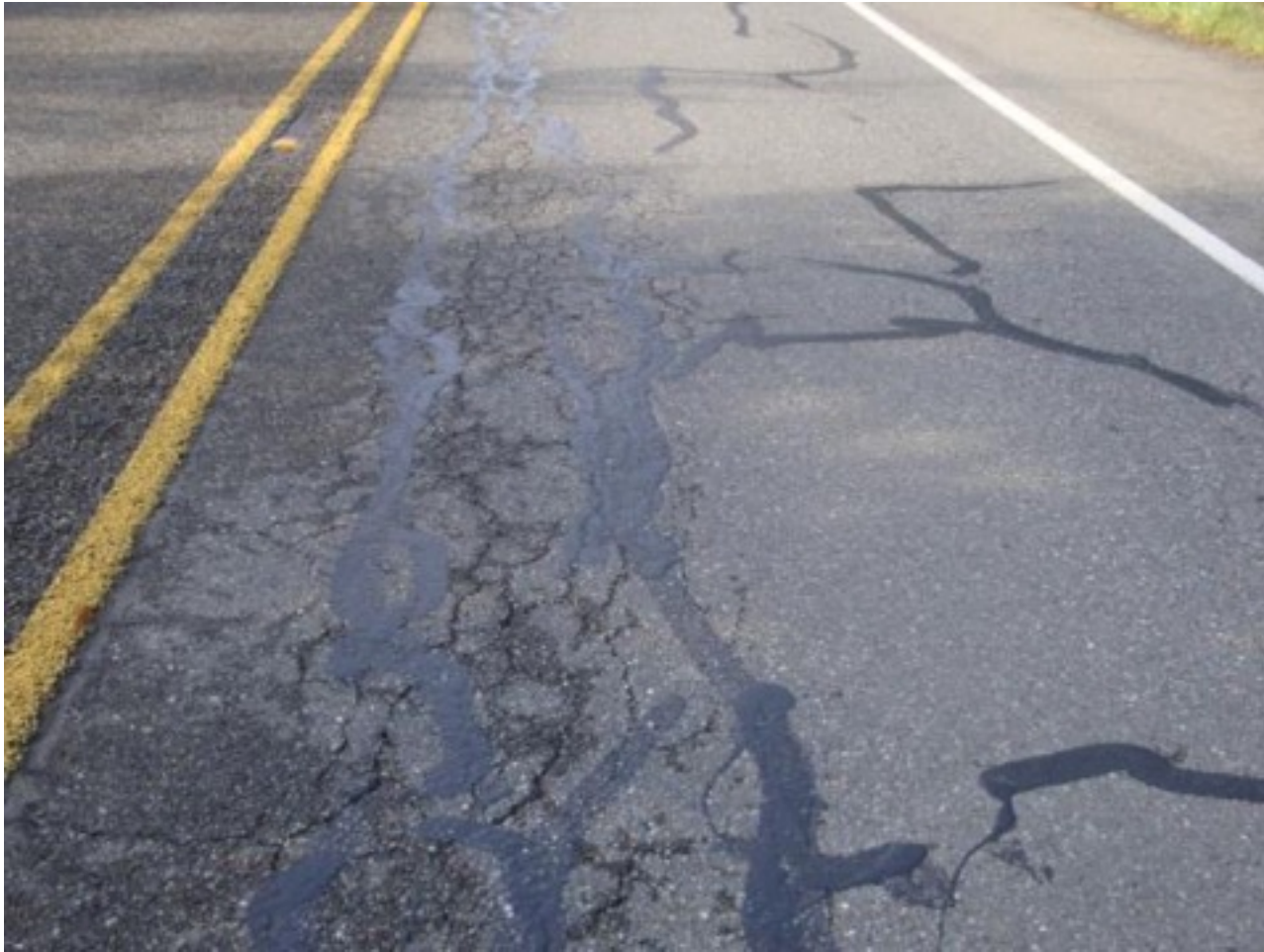
Crack sealed site after 2 years.
