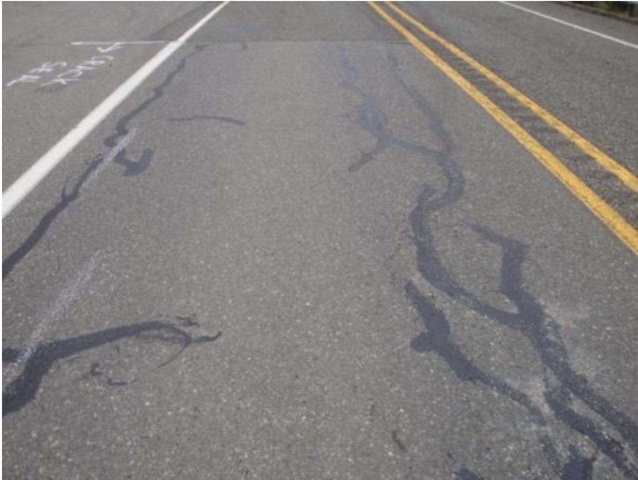
Crack sealed site after 1 year.
