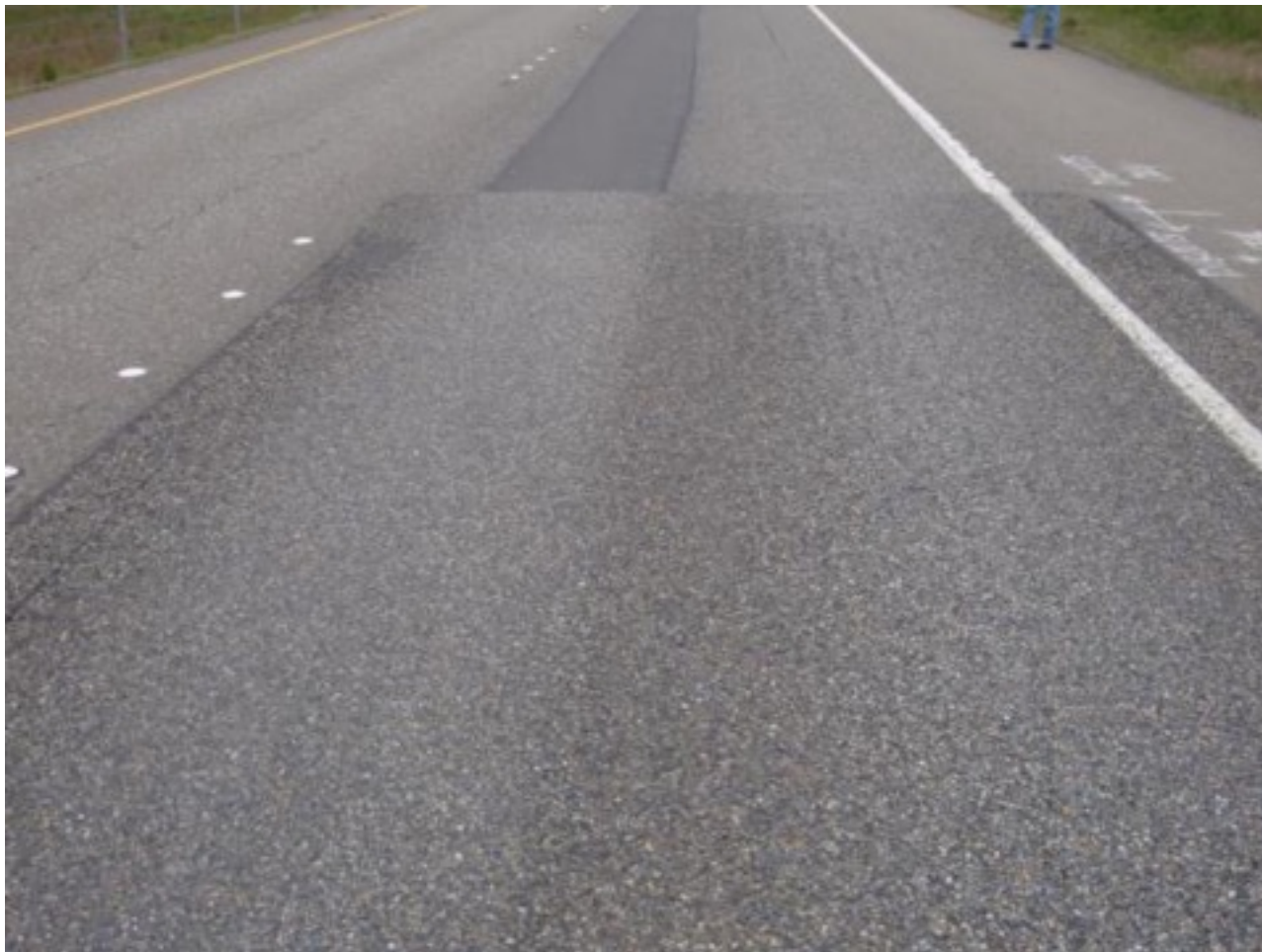
Patching and chip seal after 2 years.
