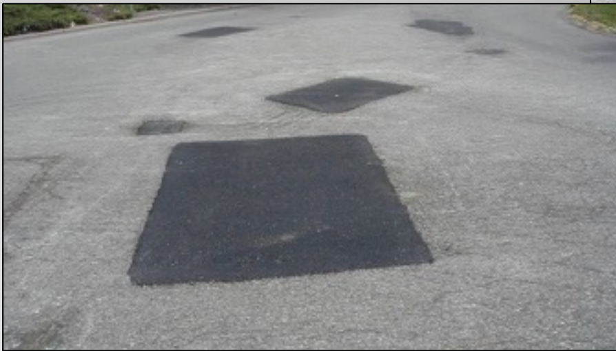
Cold compacted HMA or infrared patches
