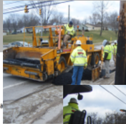
Installation using paver & roller
