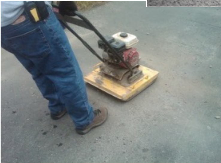
UPM mix in-place 2 years until bridge deck overlaid.
