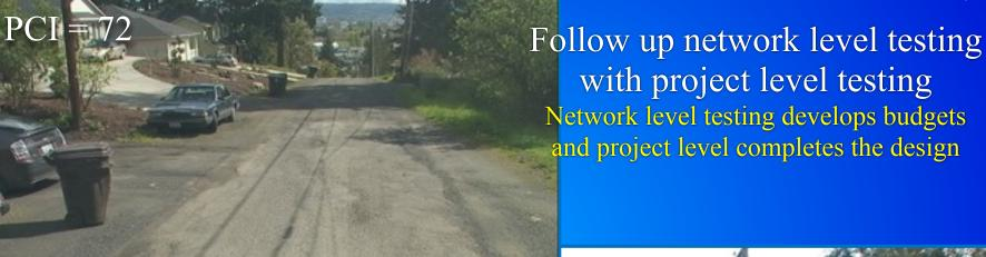
Do not assume a 2" overlay selected by the system means a 2" overlay Perform deflection testing, pull cores, and design an appropriate overlay
