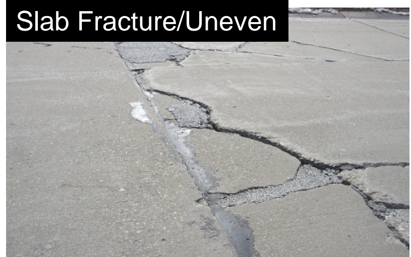
Extreme fatigue cracking/unstable base
