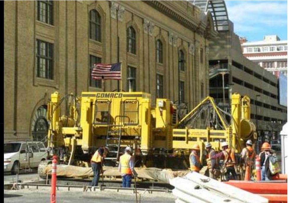
Photos from Concrete Works or Colorado, Inc. (prime contractor)
