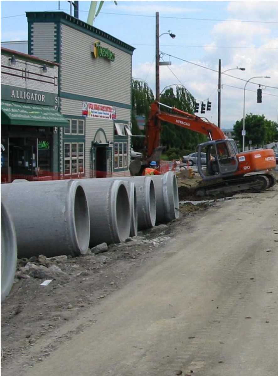
Stormwater pipe awaiting installation
