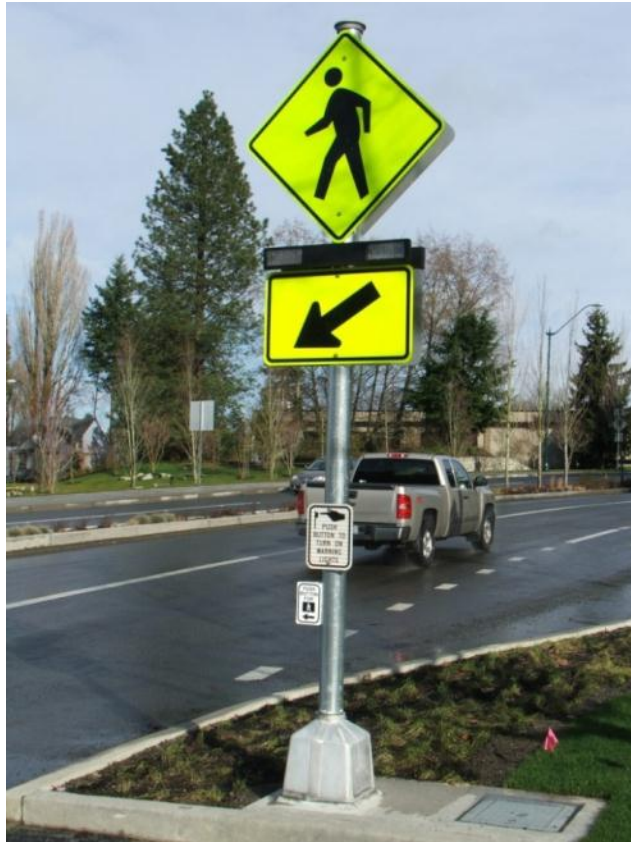
Rectangular Rapid Flashing Beacon
