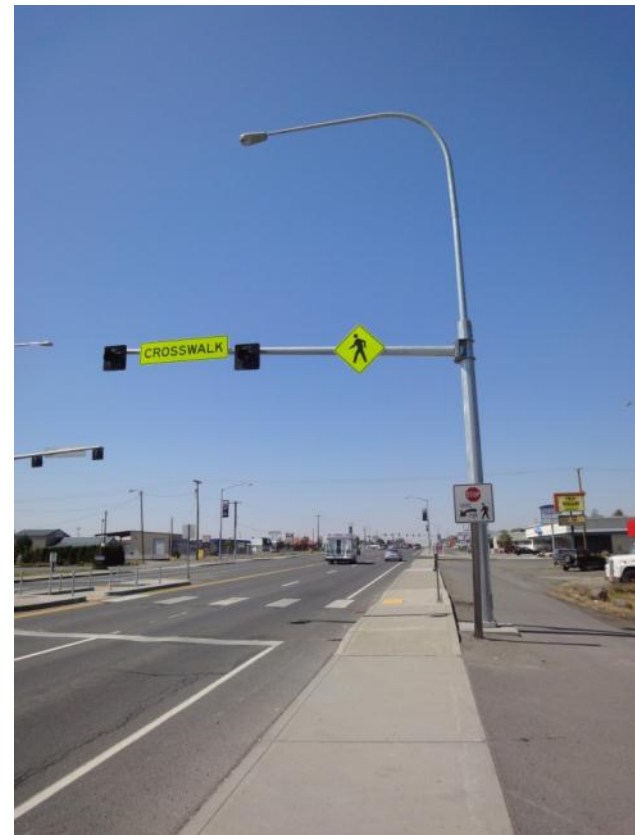
Overhead Flashing Beacon
