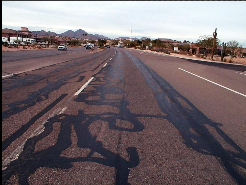
Fatigue cracking
