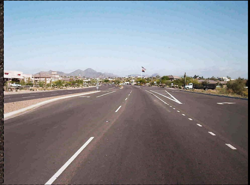
Same street- slurry seal treatment two years later
