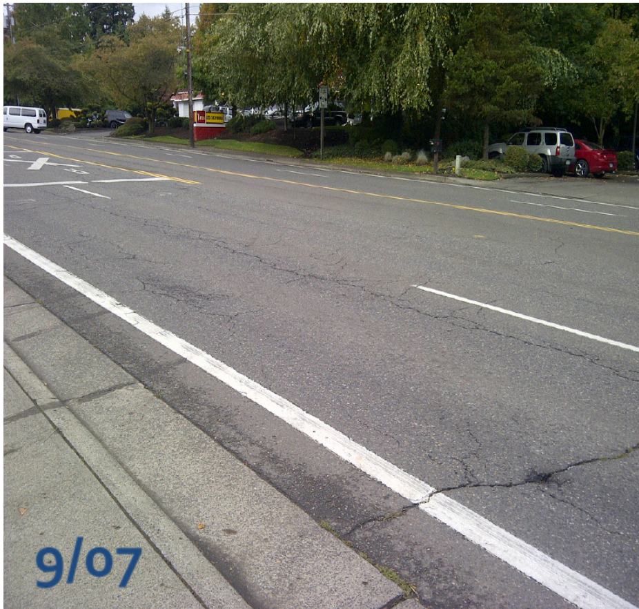
Boones Ferry - BEFORE
