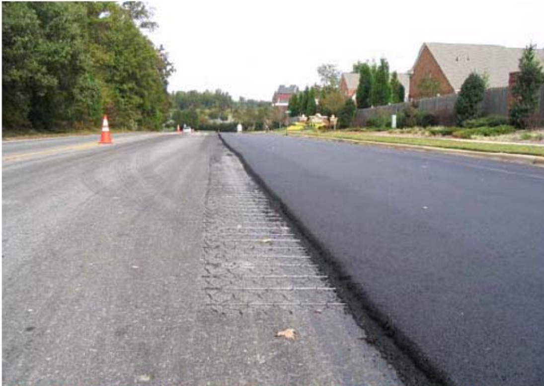
Road Mesh™ overlap to reduce construction joint cracking
