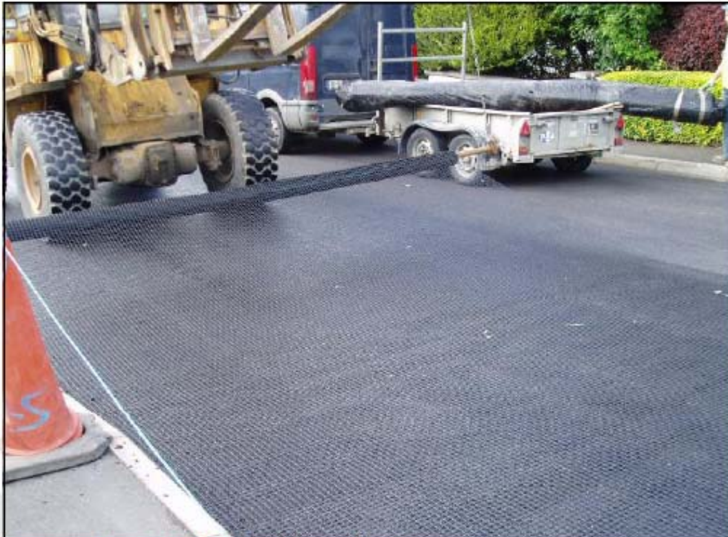
Laying MacGrid™ AR onto road surface
