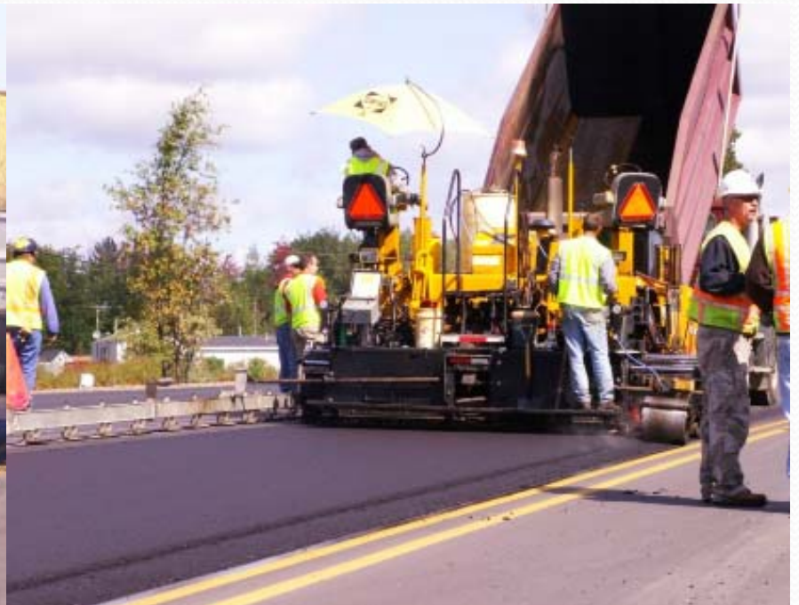
Warm Mix Asphalt
