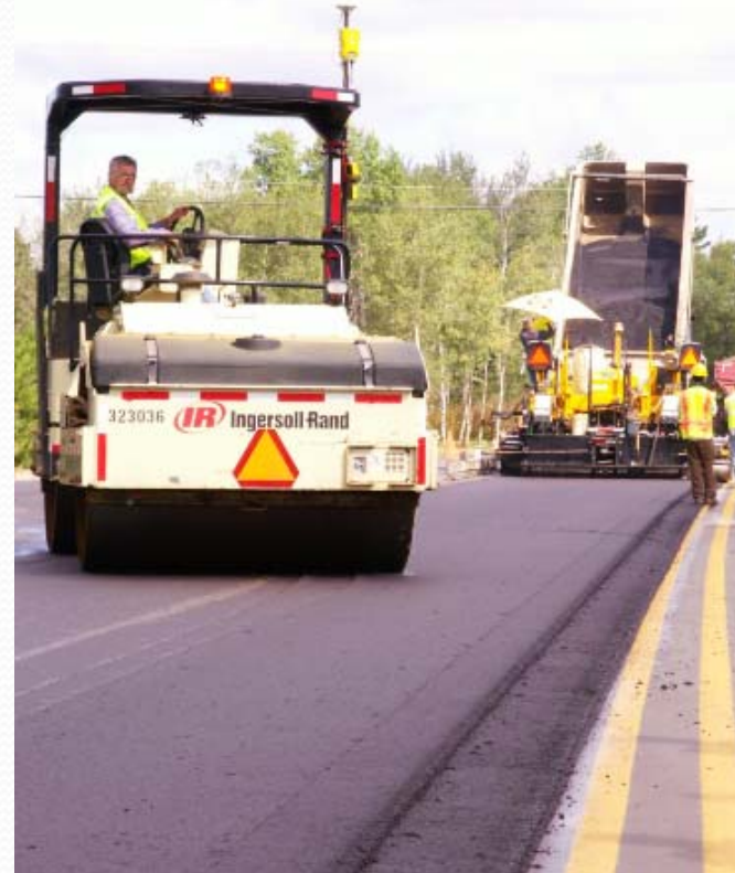
Warm Mix Asphalt
