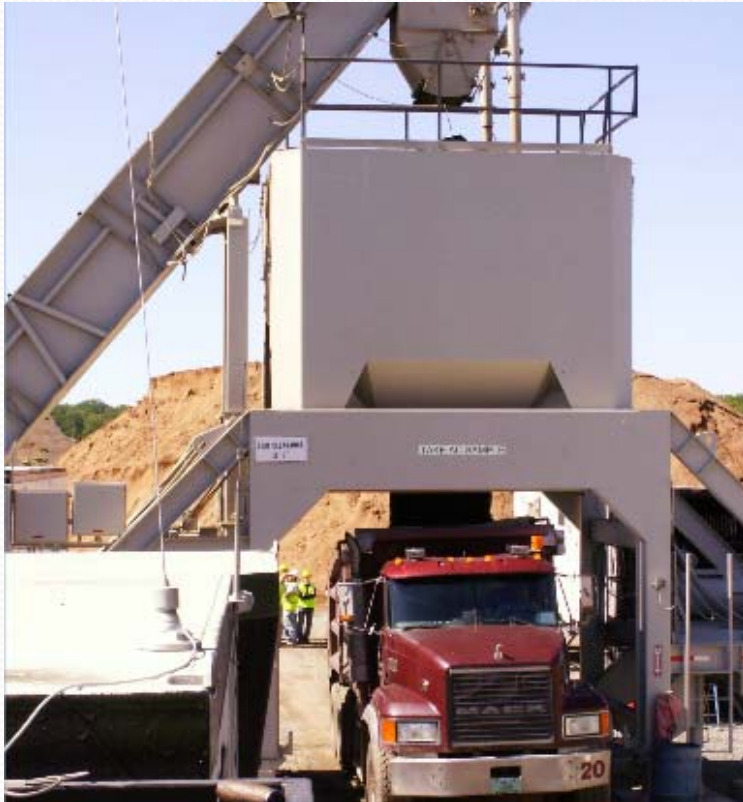
Warm Mix Asphalt
