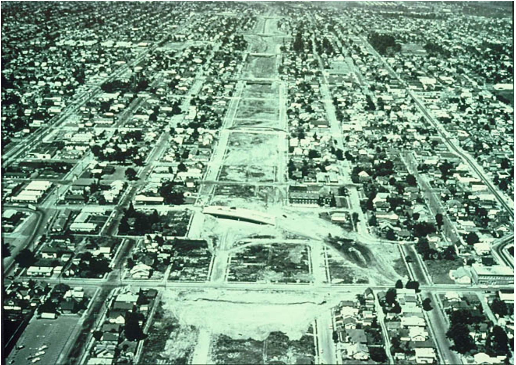
I-5 Construction through Portland in late 1950's
