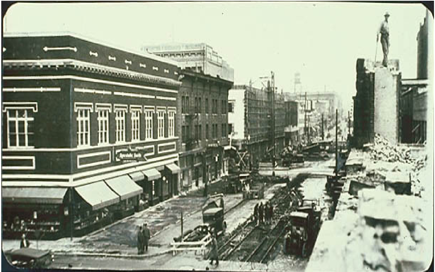
Burnside widening 1930's
