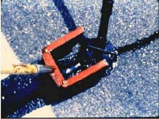
Crack Seal
