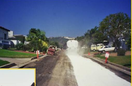
Lime application rate is determined by laboratory testing.
