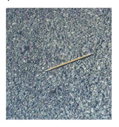
Aggregate and/or binder has started to wear away but not significantly. Appears only slightly aged and rough.
