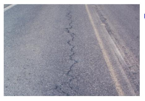
Little to no spalling and less than ¼ inch in width. If cracks are sealed they should be classified as low severity.
