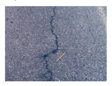
Cracks are spalled. There may be several cracks near the main crack. Pieces are visibly missing along the crack. At some point, will become alligator cracking.
