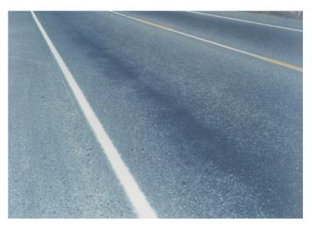
• Minor amounts of aggregate have been covered by excess asphalt but not significantly.
