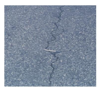
Little to no spalling but greater than ¼ inch in width. May be a few low severity connecting cracks near the main crack.
