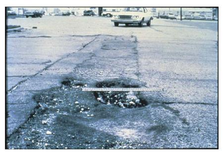
Patch has high severity distress of any type.
