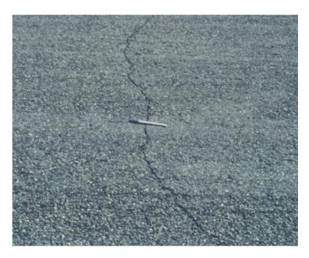
Little to no spalling and less than ¼ inch in width. If cracks are sealed they should be classified as low severity.
