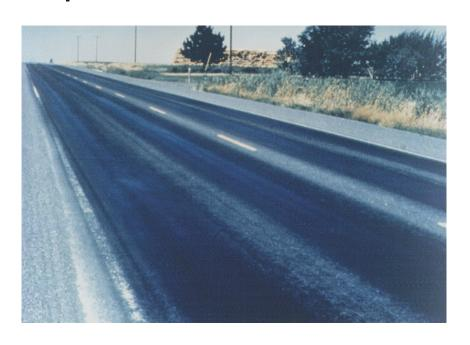
Most of the aggregate is covered by excessive asphalt. The area appears wet and is sticky in hot weather.
