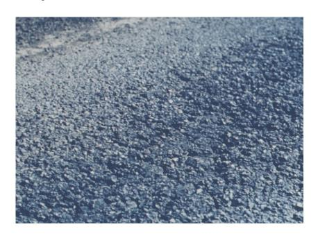
Aggregate and/or binder has worn away significantly and surface texture is deeply pitted and very rough. Fine aggregate is missing from the surface.
