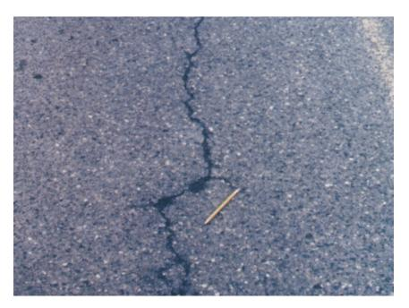
Cracks are spalled. There may be several cracks near the main crack. Pieces are visibly missing along the crack.
