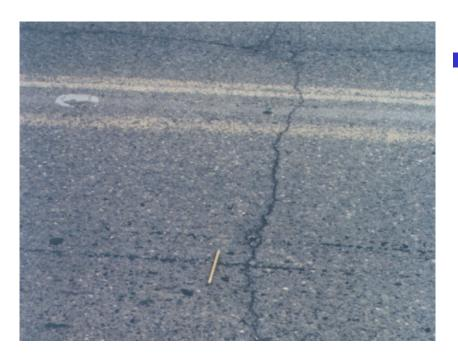
Little to no spalling but greater than ¼ inch in width. May be a few low severity connecting cracks near the main crack.
