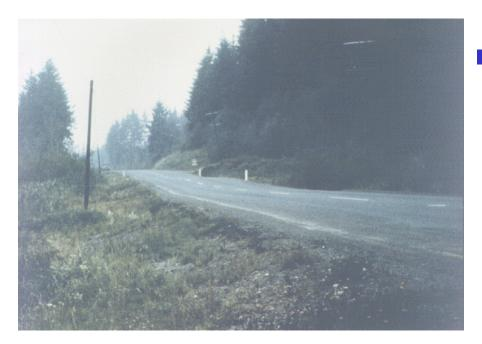
Over4 inches per ten feet. Sags and humps are defined as the maximum vertical deviation from a 10 foot straightedge along centerline.
