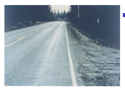
Over 4 inches per ten feet. Corrugation is defined as the maximum vertical deviation from a 10 foot straightedge along centerline.
