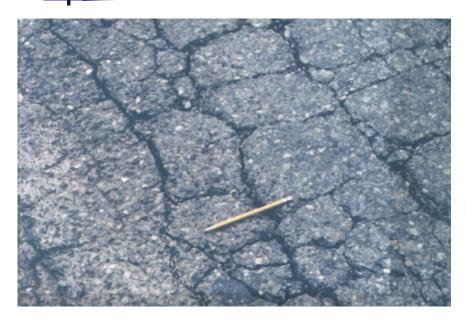
• Well developed alligator pattern. Spalling is very apparent. Individual pieces may be loose or missing. Pumping of fines may be present.
