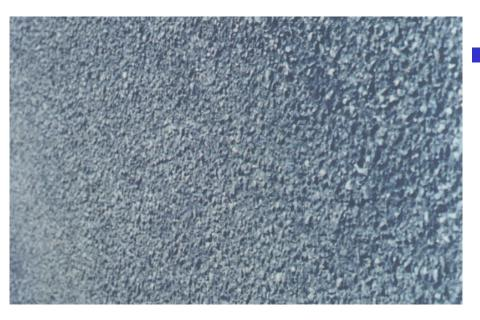
Aggregate and/or binder has worn away and the surface texture is moderately rough and pitted.
