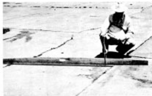
FIGURE A-10 Faulting of portland cement concrete pavement (15).
